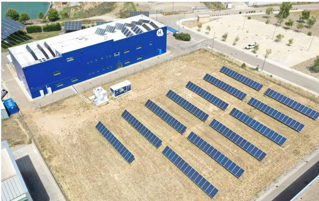
Figure 2. Aerial view of the demosite in FHa's premises in Huesca: 62 kWp of PV, 50 kW PEMWE, energy management cabinet
