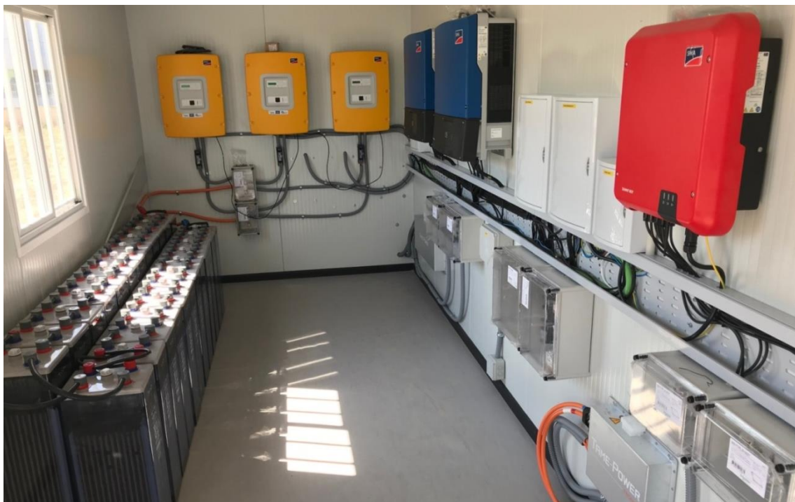
Figure 4. Inside energy management control cabinet
