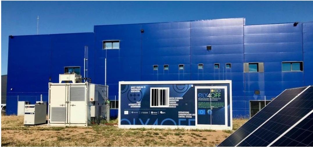
Figure 1. Demo-site (electrolyser on left, energy management system on right)
