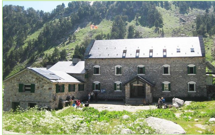
Figure 7. Off grid mountain installations
