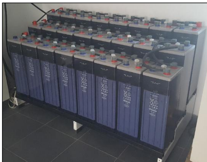
Figure 10: Lead-Acid batteries which will be used for ELY4OFF project
