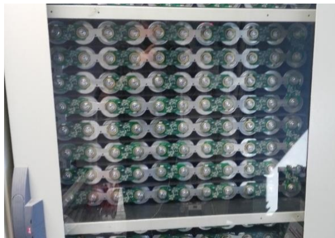
Figure 25. Demo installation of Supercapacitors for UPS
